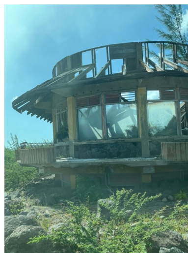
Top floor of a four-storey building.
